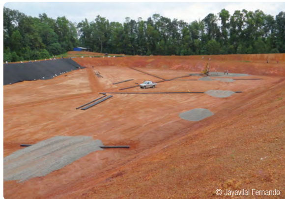
Sanitary landfill under construction , Sri Lanka
