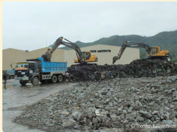
Temporary dumpsite, Tacloban Abucay
