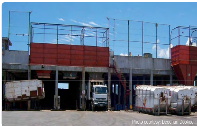
A transfer station in Mauritius
