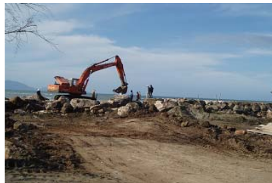
Construction of sea wall in front of aquaculture ponds in Lham Dingin village (Photograph: Suryadiputra, September 2005)
