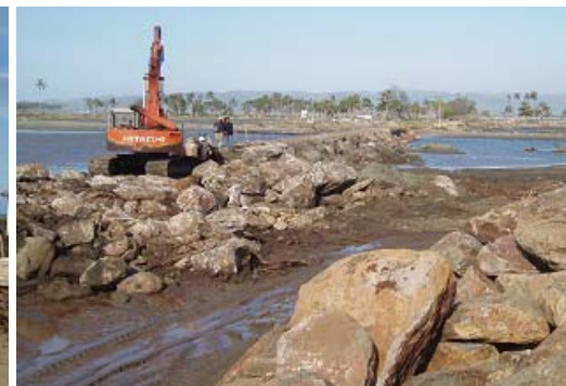
Construction of sea wall in front of aquaculture ponds in Lham Dingin village (Photograph: Suryadiputra, September 2005)
