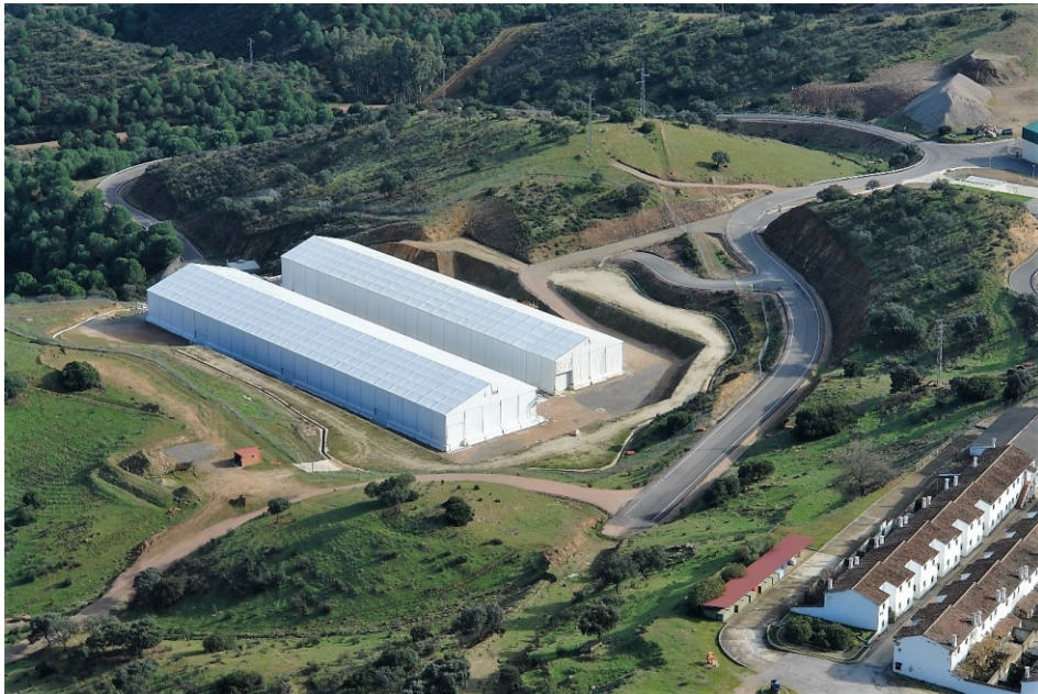
Image of the LILW disposal cells at El Cabril.
