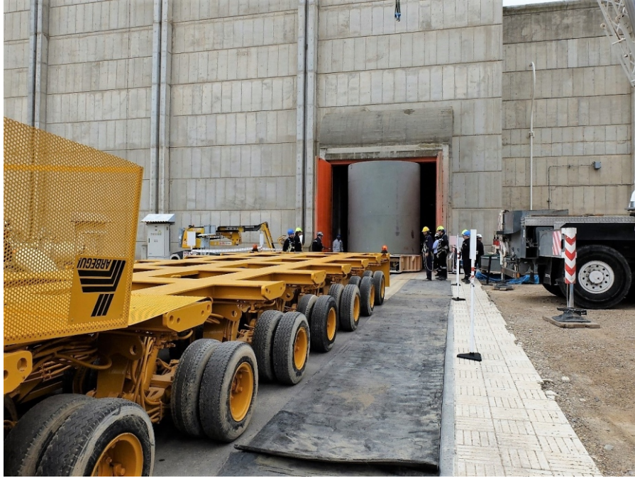
Image of the removal of the loaded cask from the Ascó fuel building
