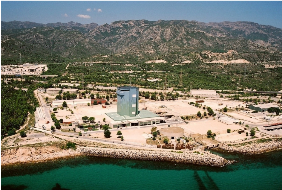
Image of Vandellós 1 nuclear power plant in dismantling phase. It is currently in the latency phase.
