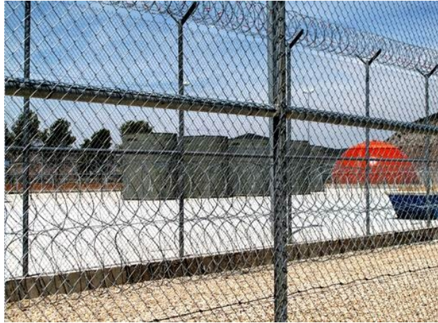
The José Cabrera Nuclear Power Plant ISFSI facility.
