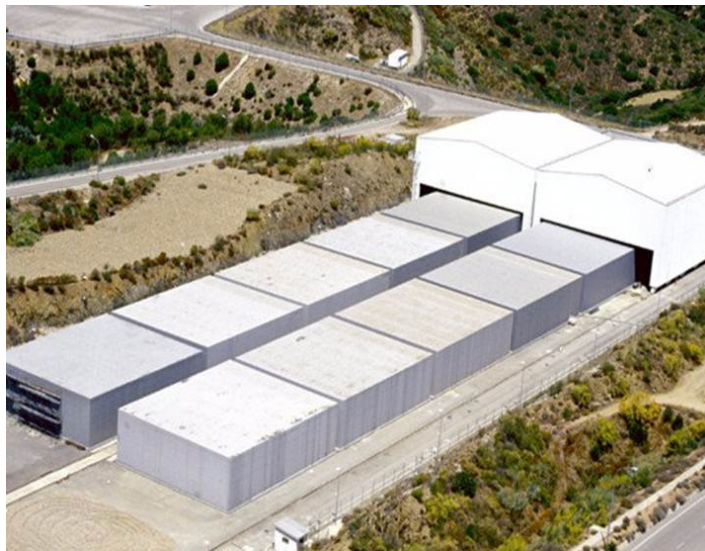
LILW vaults at ENRESA's El Cabril disposal facility.
