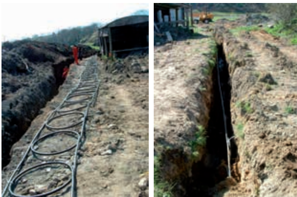
Figura 6.7: Slinky vertical
