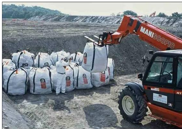
Figure 1.5-2: Disposal of asbestos waste at the landfill site Villeparisis (France)
