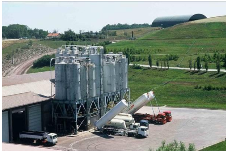
Figure 1.5-3: Stabilisation plant of the landfill Villeparisis (France)
