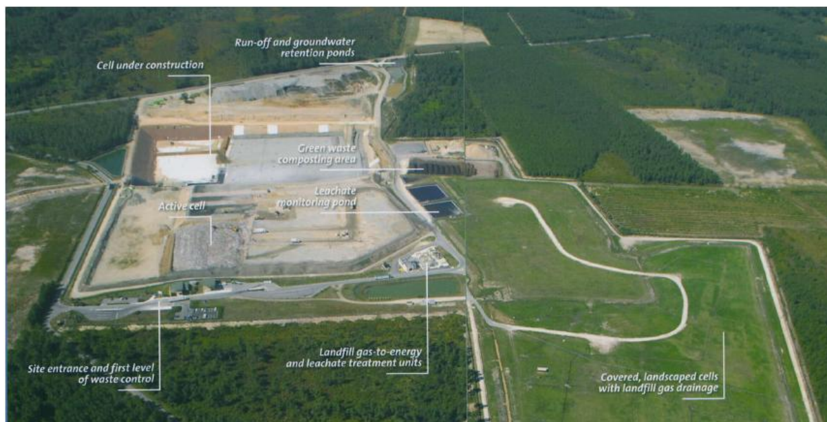
Figure 1.5-8 : Aerial view of Lapouyade class B landfill site
