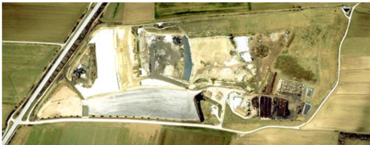
Figure 1.1-1: Overview of Langenlois Landfill (Austria)
