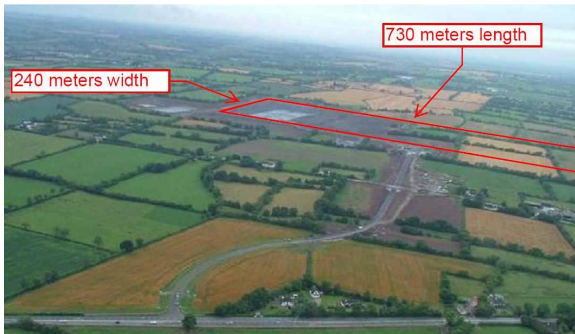
Figure -1.8-2: Overview of the landfill Greenstat at Knockharley (Ireland)
